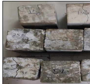
Fig. 6 Concrete cubes cracked after 28 days
